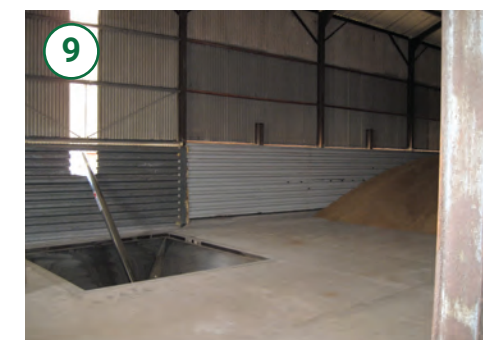
9 Reception pit allows tipping straight from the field or filling with the handler from a wet grain heap.
