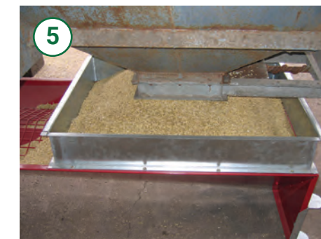
5 An adjustable sluice that controls the flow of grain is required with some designs of pre-store hopper.
